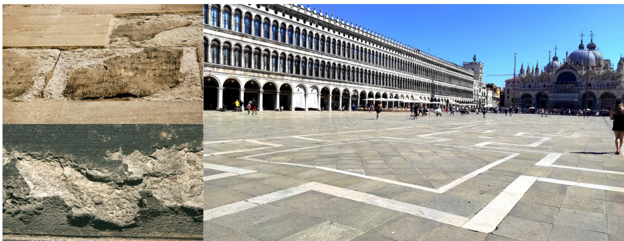
Figure 2.4: Left: Typical disintegration and flaking of trachyte stone [60]. Right: San Marco square, Venice, a world renowned symbol paved with Euganean trachyte.
